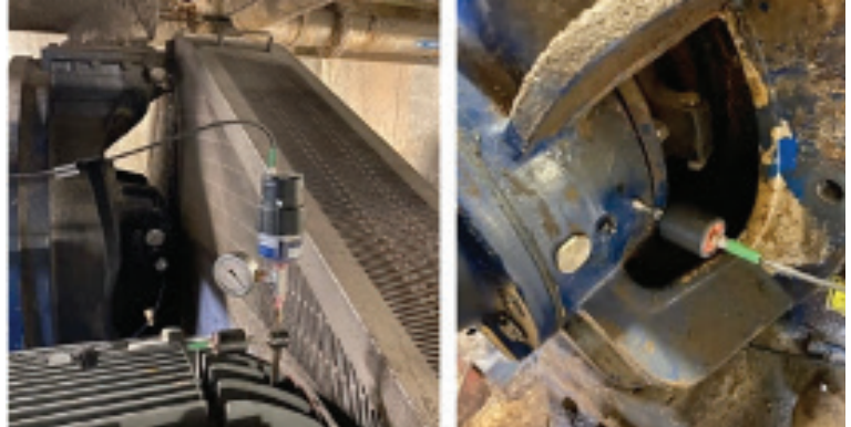
Figure 15: ON-GUARD Installation DE & NDE
